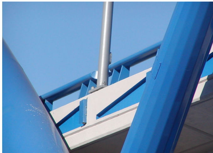
TxDOT T4(S) Mod Painted Arapaho Road Bridge, Addison, Texas
