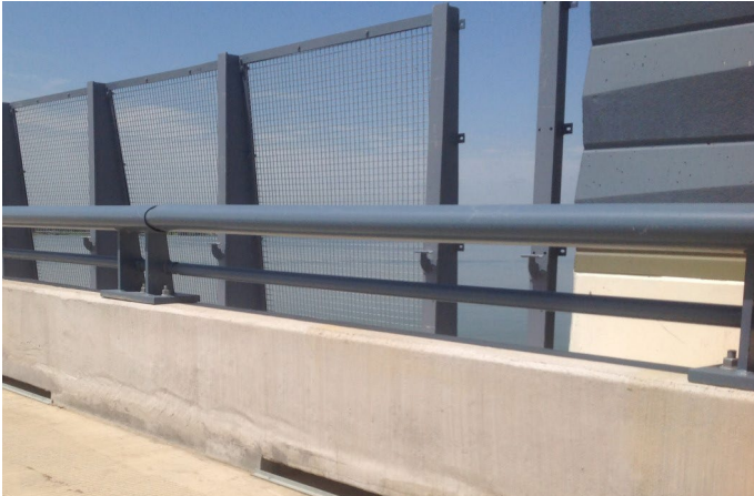
TxDOT C402 Painted TL-3 Lake Lewisville Bridge, Lewisville, Texas
