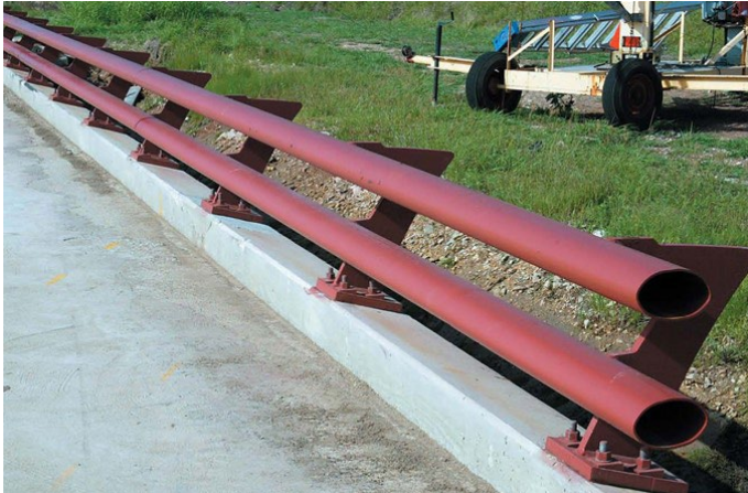
TxDOT T77 TL-3 TTI Test Center, Texas A&M University
