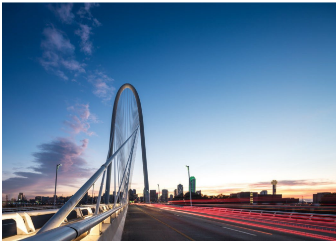
TxDOT HT TL-5, Designed by Santiago Calatrava Margaret Hunt Hill Bridge, Dallas, Texas
