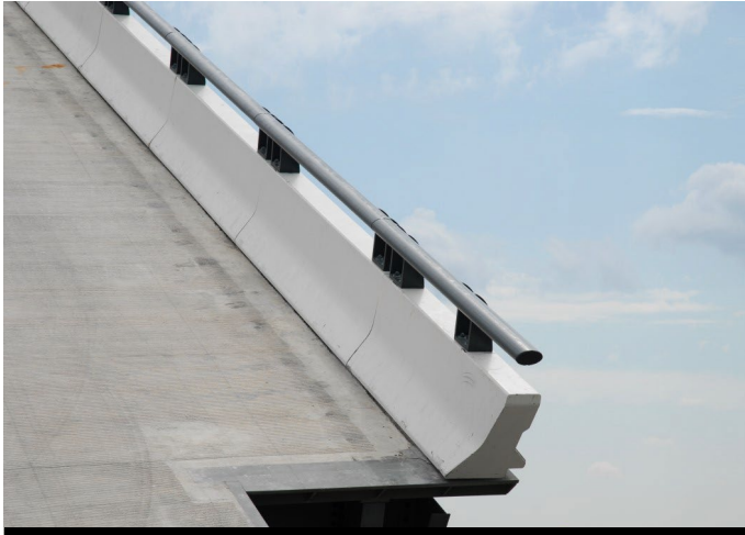
TH80 (TL5) on I-95 over Potomac River Woodrow Wilson Memorial Bridge, Maryland
