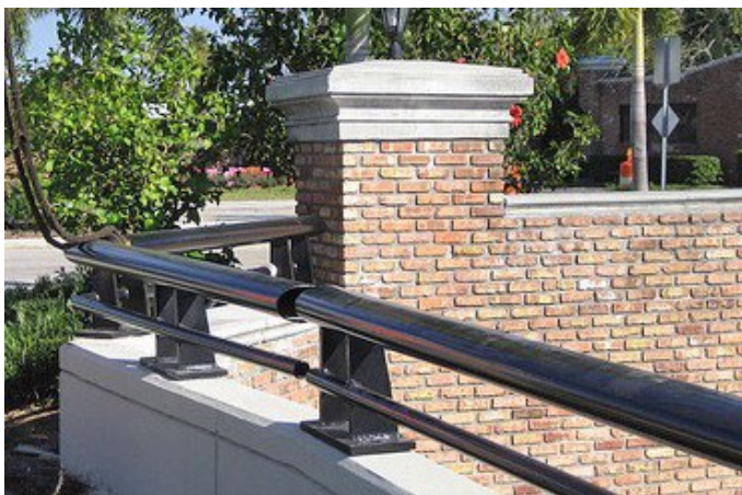
FDOT C402 Painted (TxDOT Standard) Preserve Golf Course, Plantation, Florida
