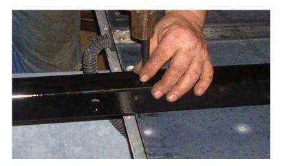
c. Attach the bottom of each support tube with a 3/8"x6" grade 5 bolt, nut, washer, lock washer, and 2-5/8" long, 5/8"x1/16" sign mounting sleeve.
