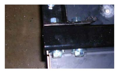
b. Mark the bolt hole locations on the bottom of the sign panel with a center punch. Drill one 7/16" hole in the base of the sign panel to attach each support tube.Make sure the hole in the bottom flange of the sign is aligned with the hole in the top flange.
