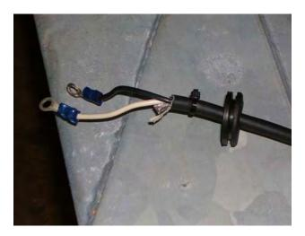
e. Place the conductor in the box with the seal in its seat. Connect the hot wire to the blue pole, the pole at the front of the box. Connect the ground wire to the white pole on the rear of the box. Make sure wires do not obstruct the screw sockets used to attach the top of the junction box. Replace the wire nuts.
