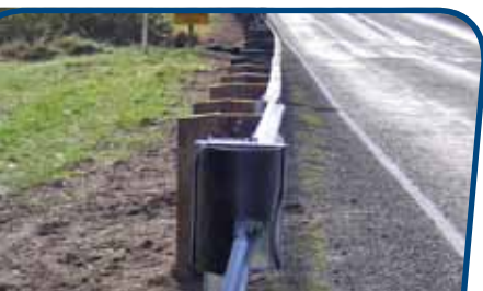
The X-Tension Terminal can be installed either flared or tangent.
