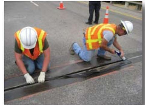
The Silicoflex System consists of an inverted 'V' shaped, preformed, extruded silicone rubber seal, with a single component silicone locking adhesive and a primer. Two beads of silicone locking adhesive are used; one above and one below the silicone rubber seal to ensure a tenacious, water-tight and continuous seal.
